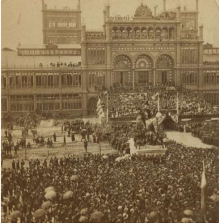
Opening day of the 1876 Centennial Exhibition in Fairmount Park, Philadelphia (Centennial Photographic Company, Public Domain)
